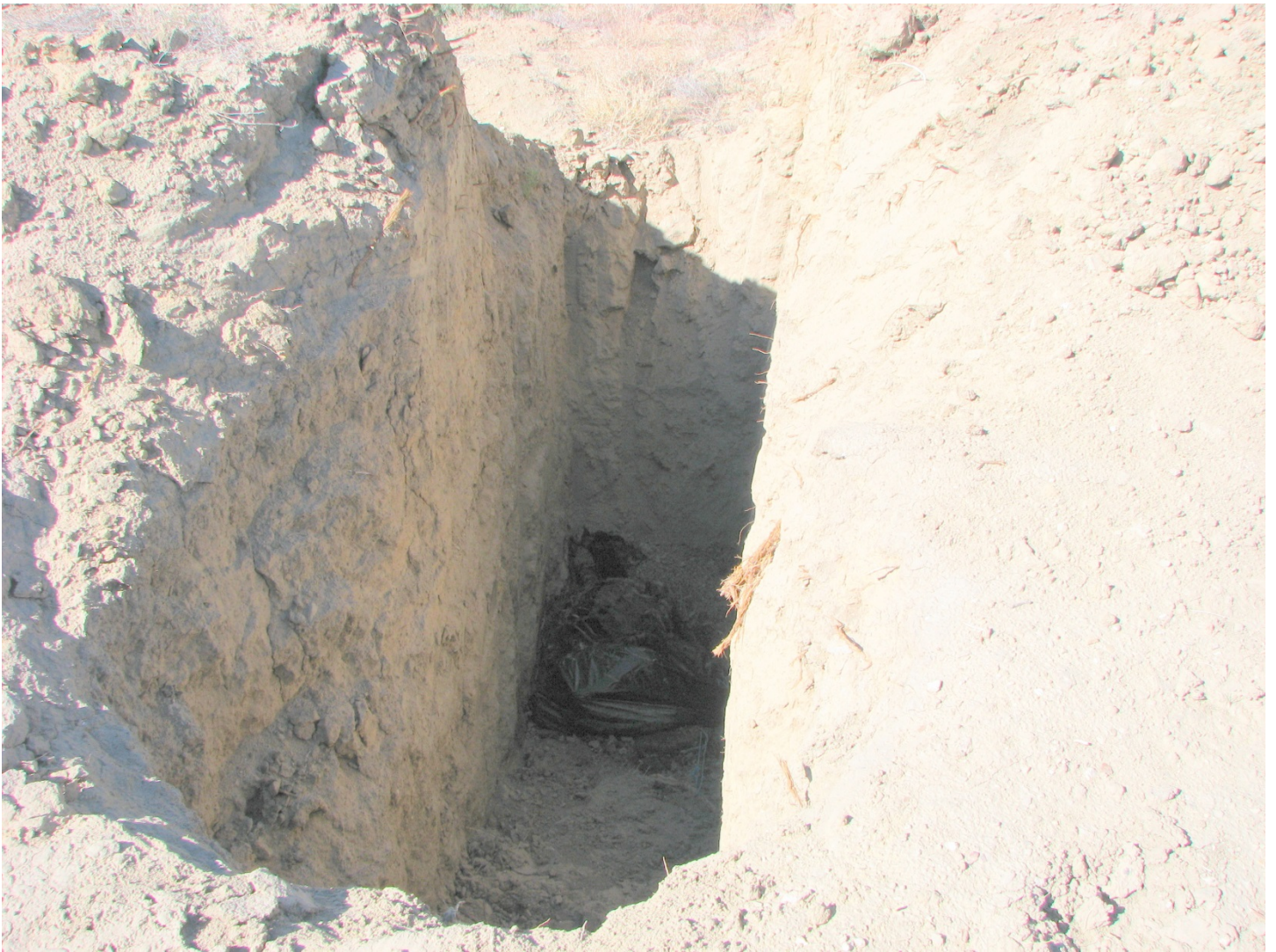
An animal carcass that has not been covered. Cover should be placed over the animal at the end of the day.
